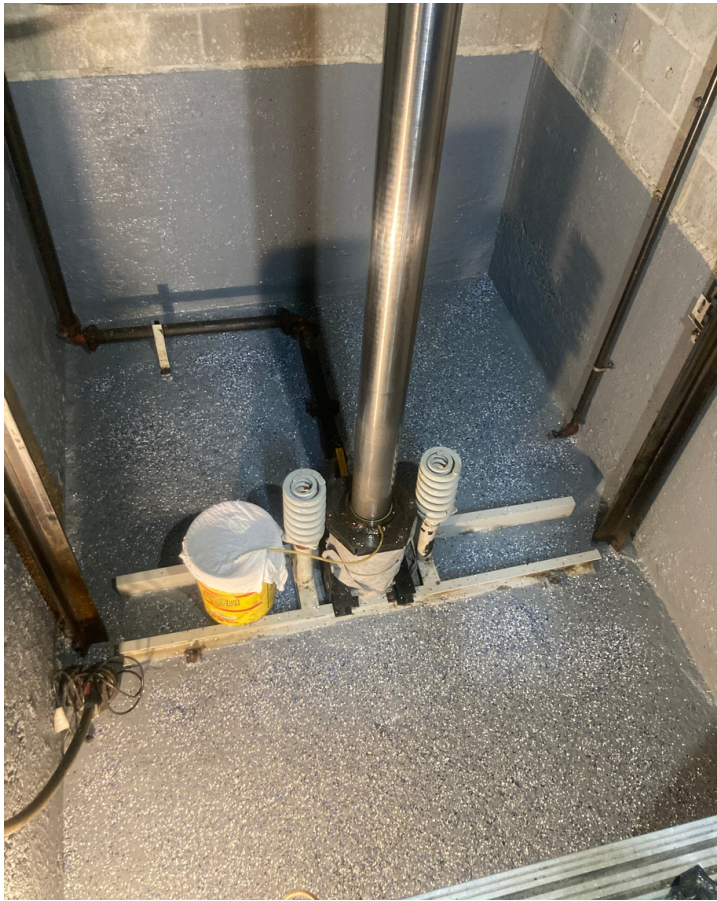
Elevator 2 waterproofed & painted
