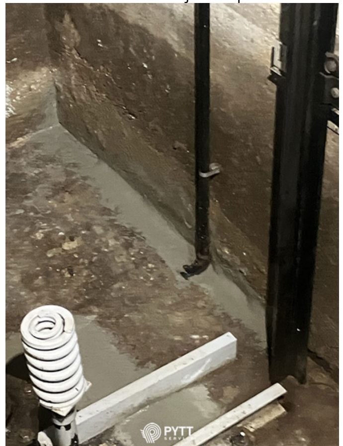
Right wall seam
