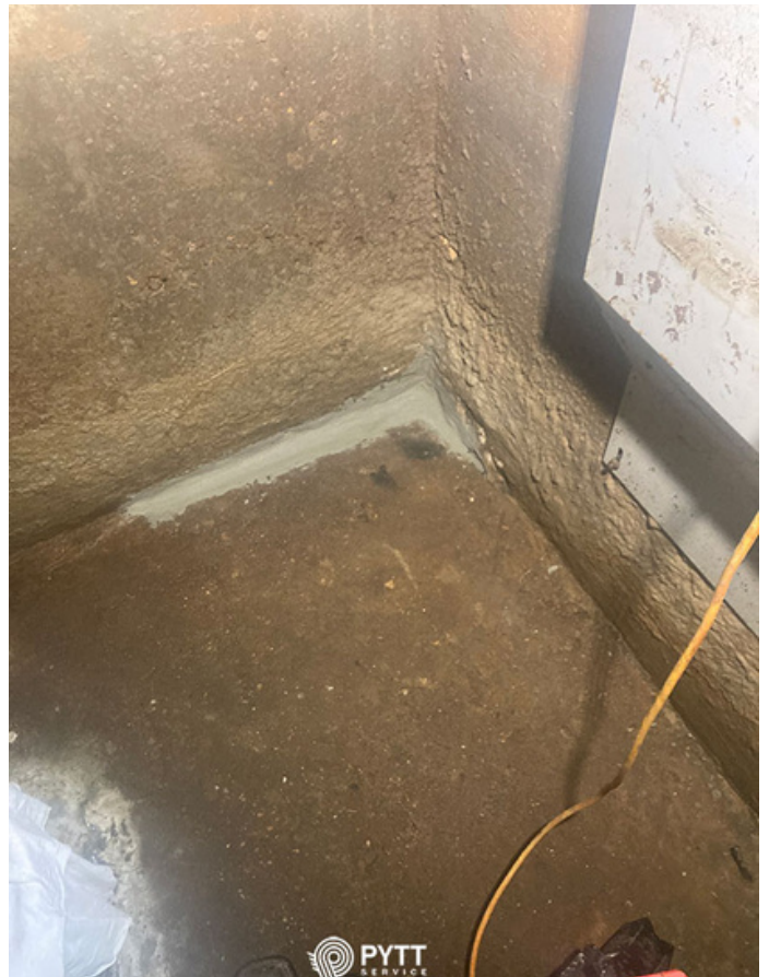
Door-side waterproofing (R)
