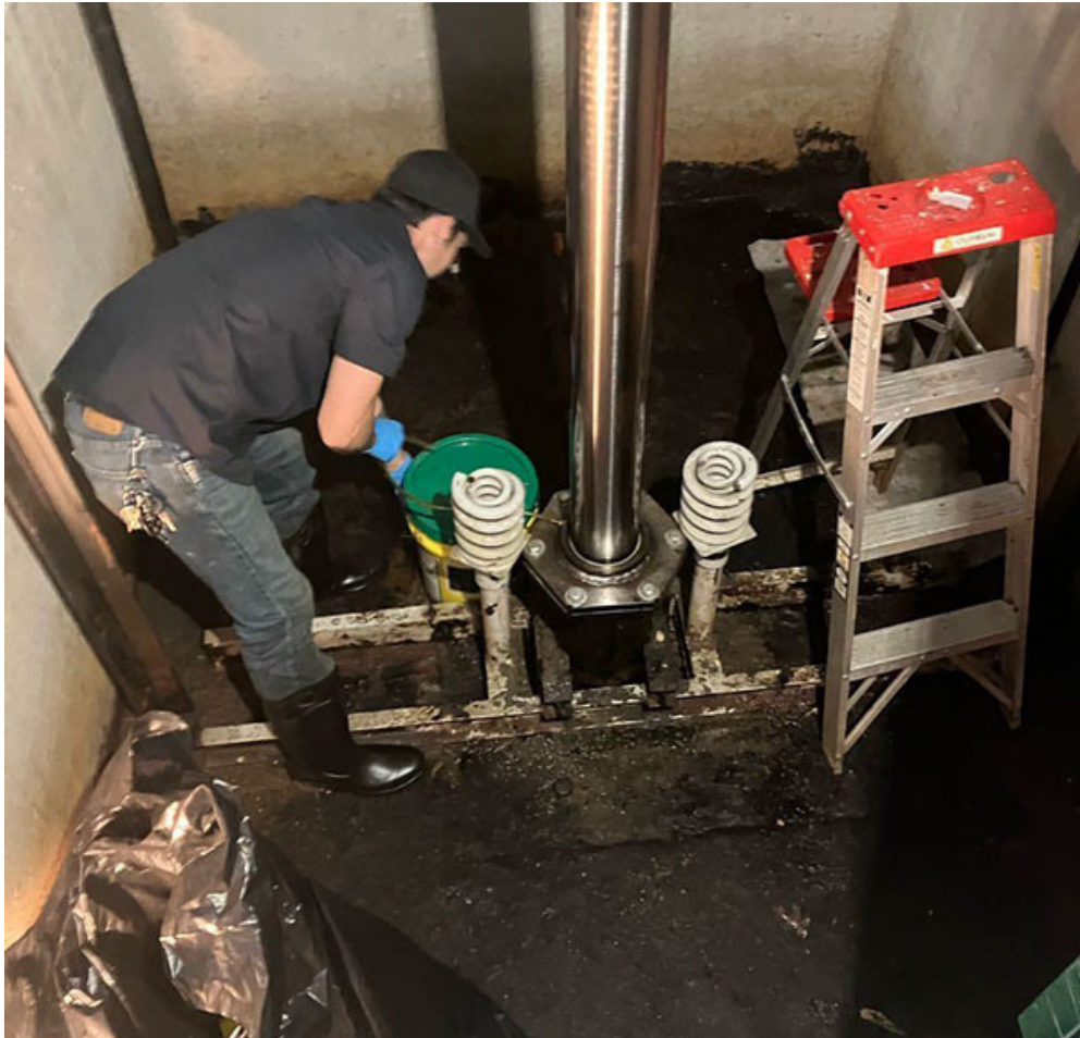
Site cleanup & de-greaser application
