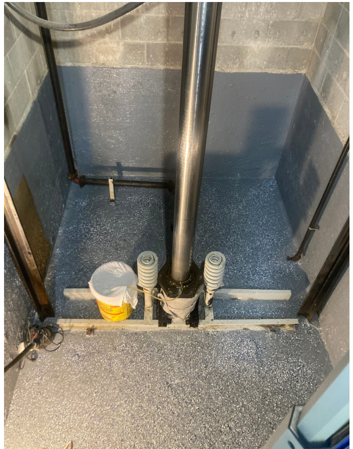
Elevator 2 waterproofed & painted
