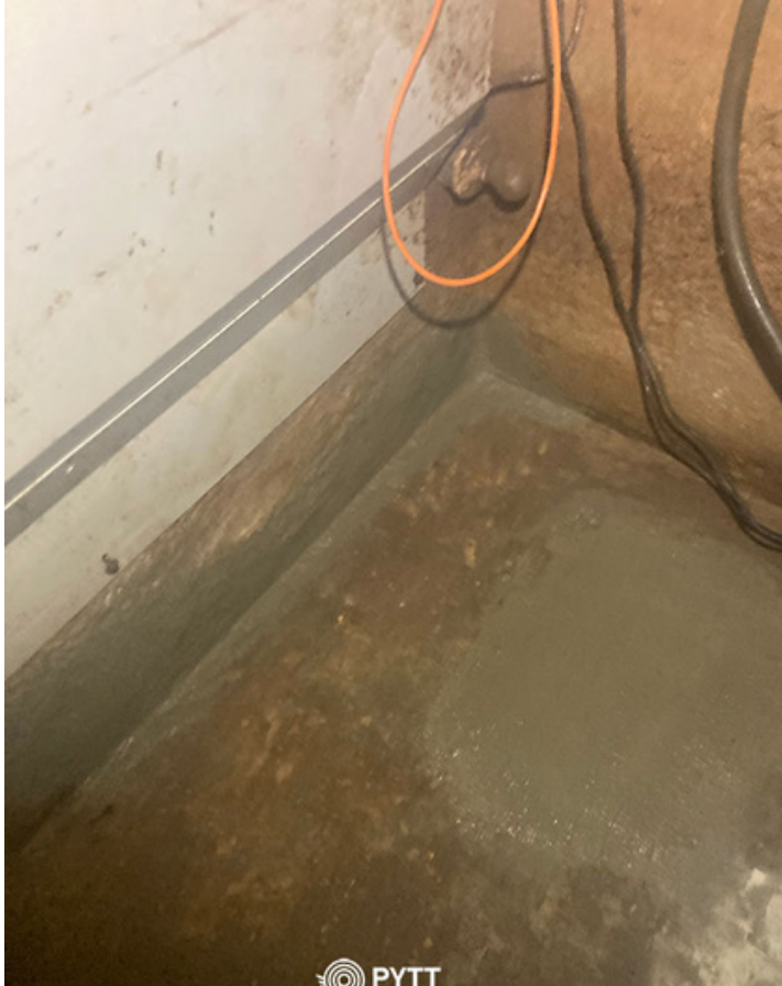
Door-side waterproofing (L)
