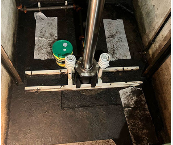
Cleaned up the elevator pit, removing all debris and oil buckets, and pressure washing.
