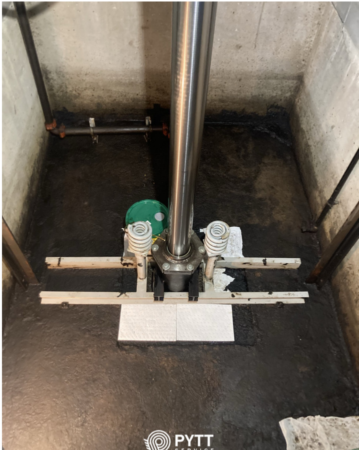
Elevator 1 Oil Pumped Out
