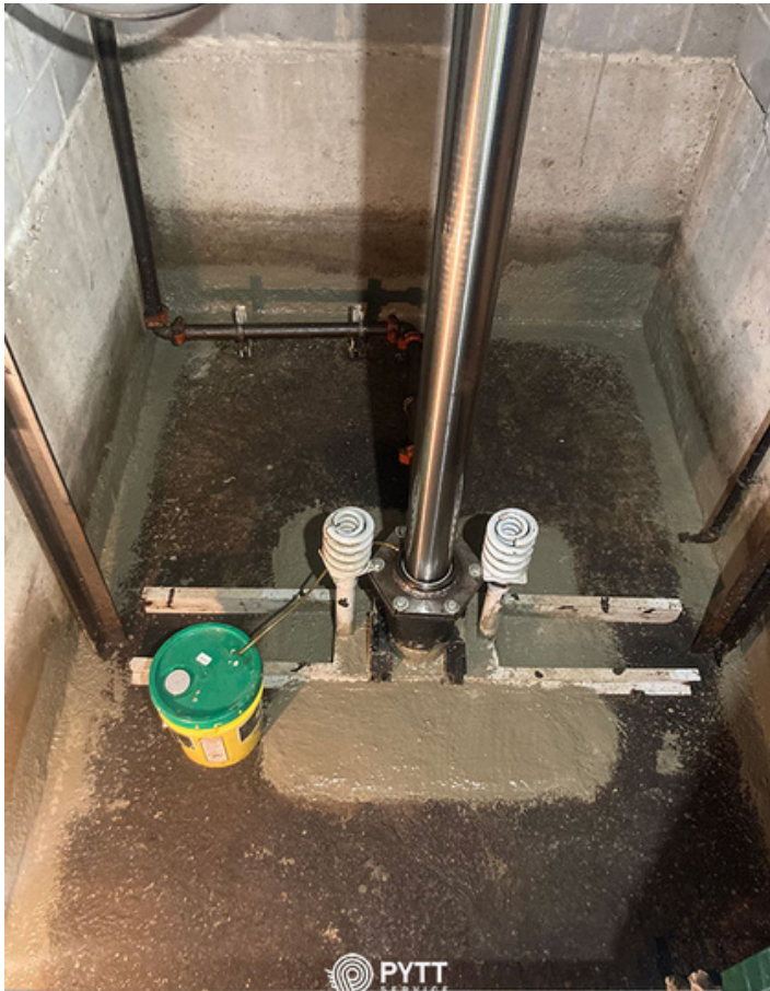
Second layer of waterproofing applied.
