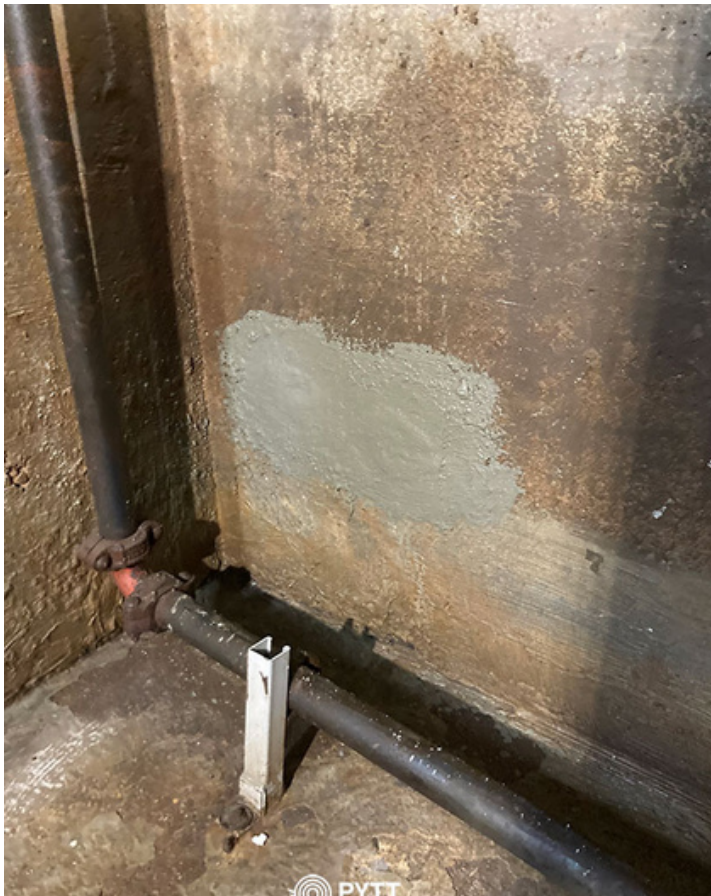
Back wall void waterproofing
