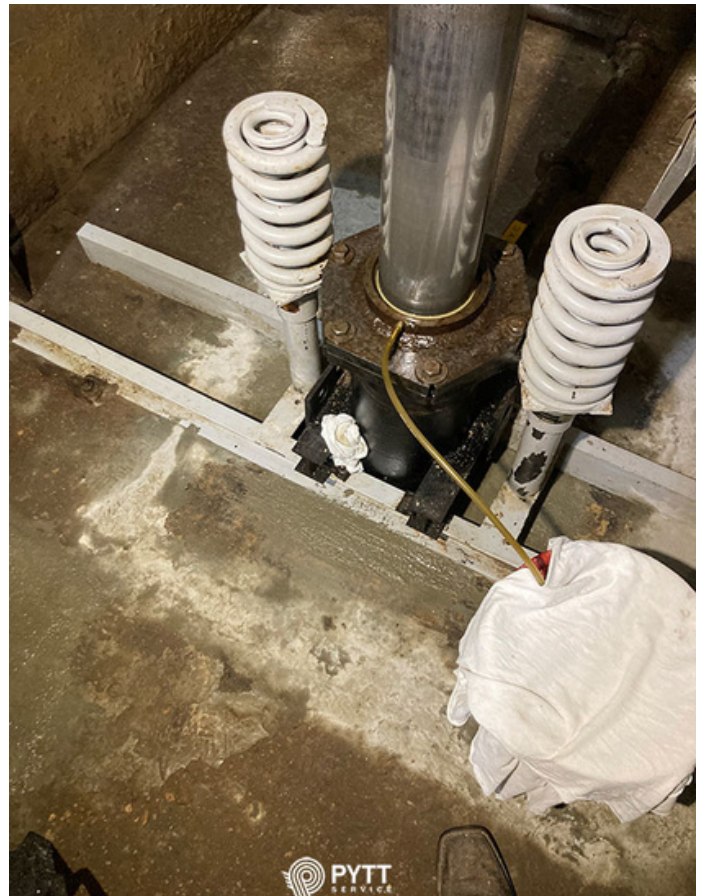
Jack cap waterproofing
