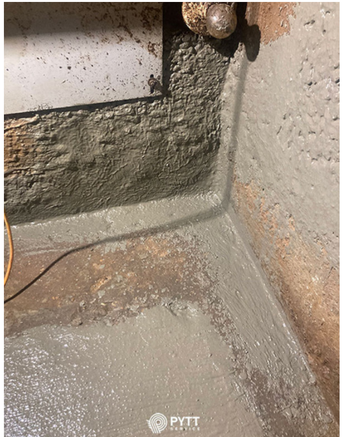
Waterproofing coat over corner
