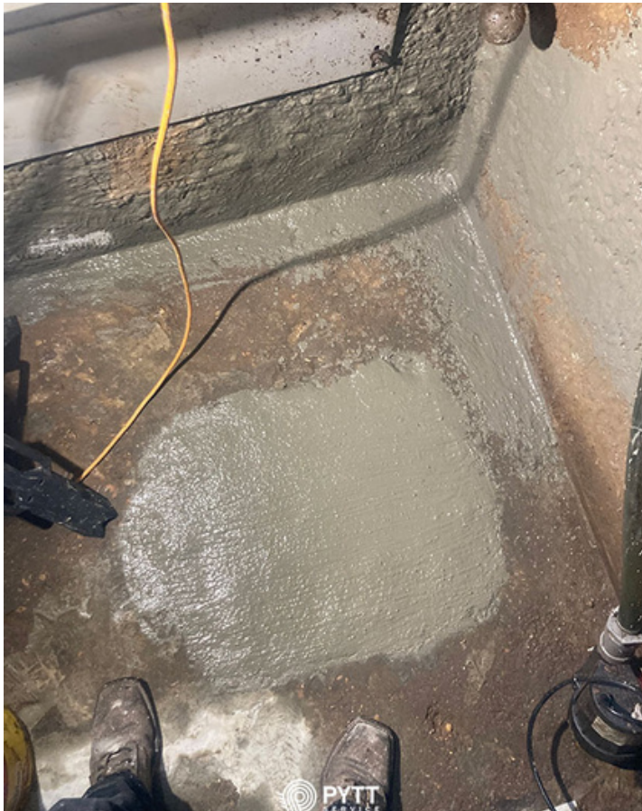
Waterproofing coat over channel fill
