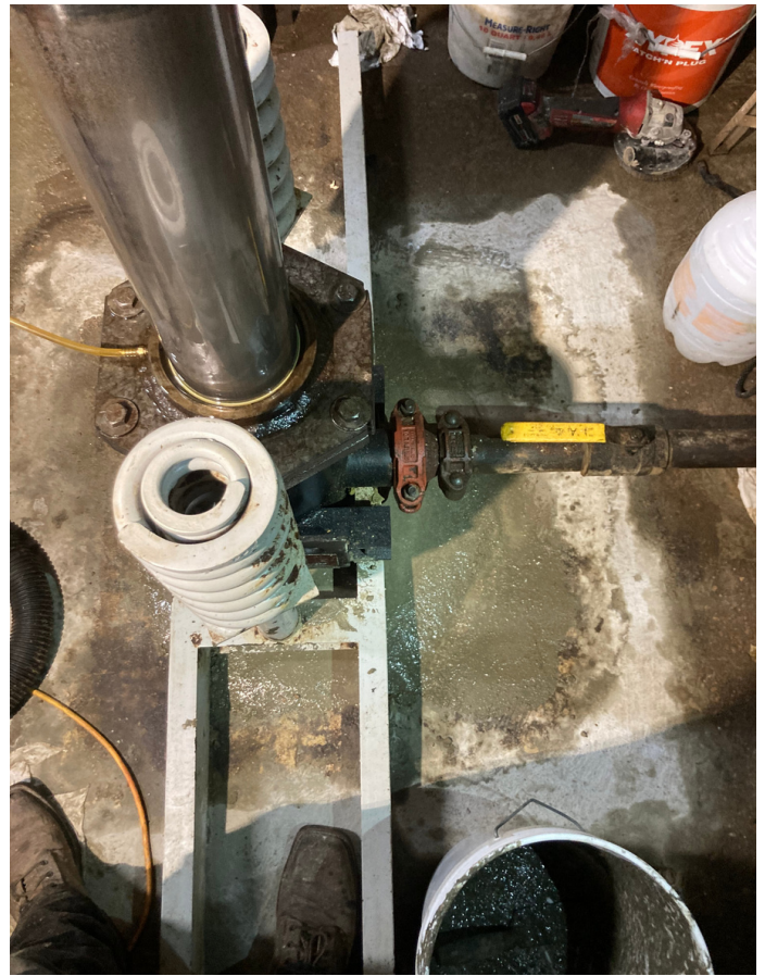
Jack cap waterproofing
