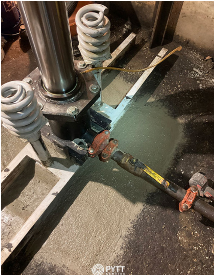
Elevator 1 Jack Cap Replacement, First layer of waterproofing applied
