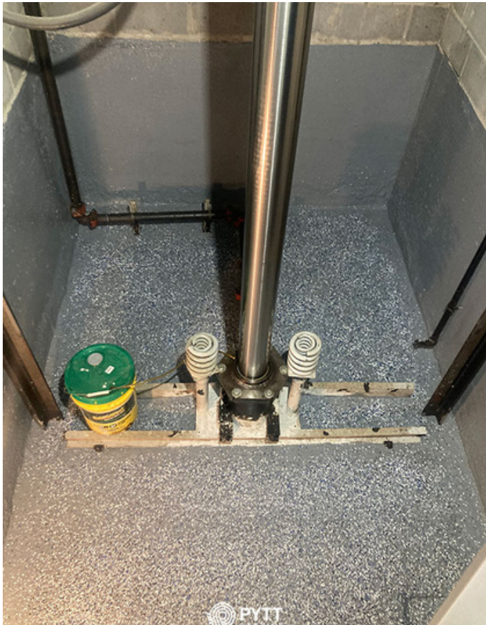
Elevator 1 elevator pit painted and finished
